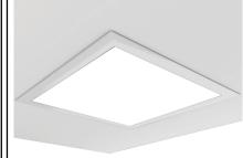
Once clips have been folded up, push panel up flush to the ceiling, Clean off any fingerprints left behind.
